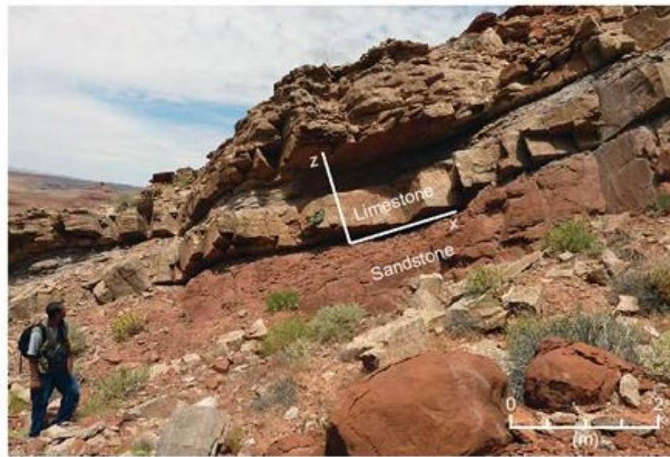
Figure 3.10 A prominent limestone bed (gray) overlies a sandstone bed (red) on the western limb of Raplee anticline, UT. The bedding interface is a discontinuity in mass density that could be explicitly defined when building a structural model at this scale. Approximate location UTM 12 S 603875.00 m E, 4115539.00 m N.
